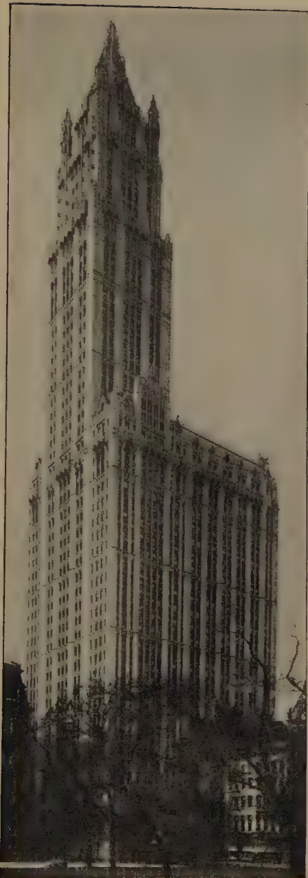
467 Cass Gilbert, architect; photograph by Wurts Brothers
